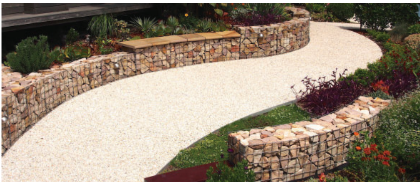
Terraced Seating, Gabion Basket Retaining Features
